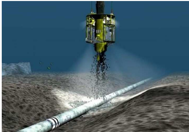
Fig. 12.1-3 Ramming of subsea pipeline in deep water area
